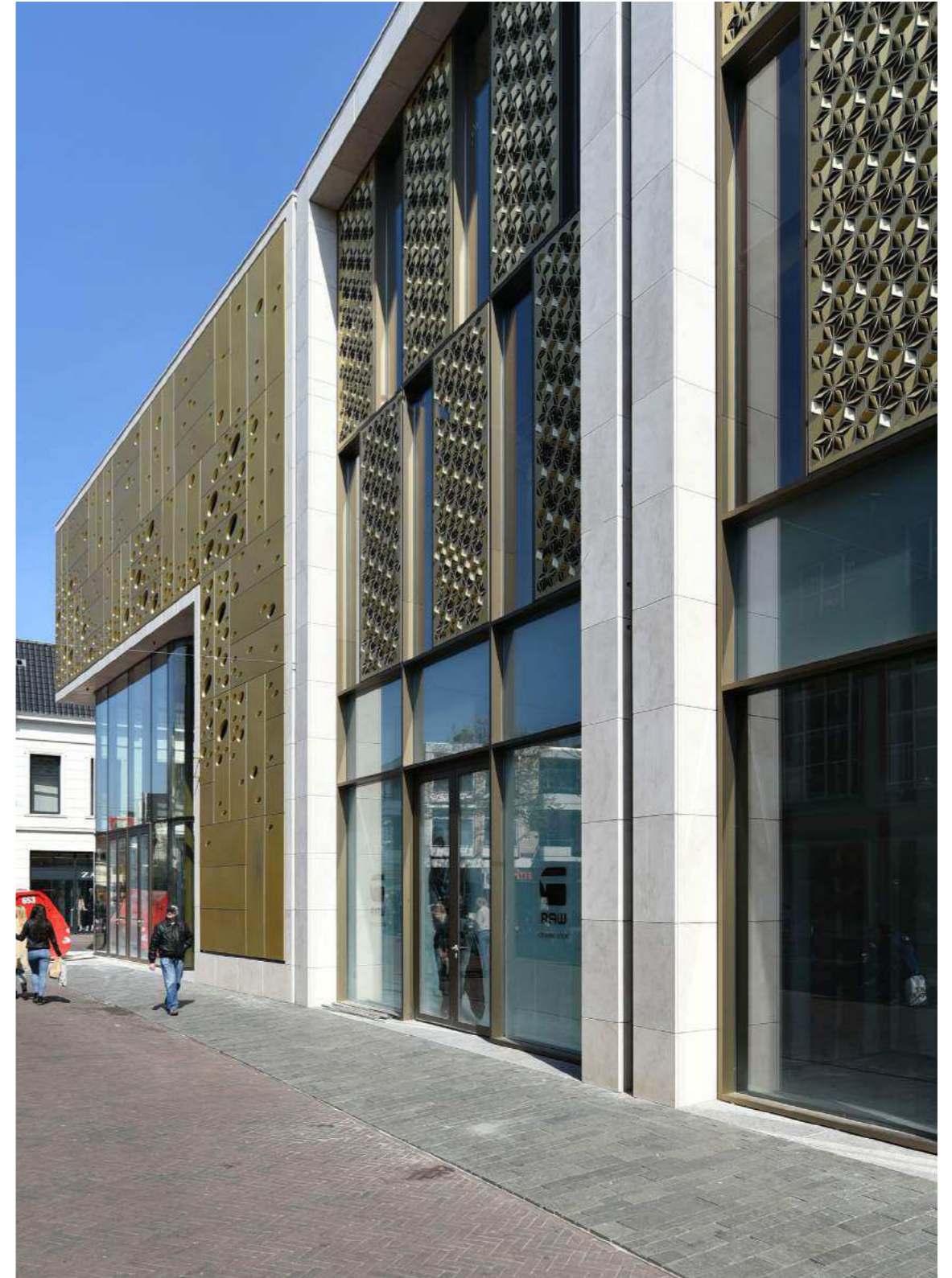
With MD Resto the panel attachments are concealed on the back side of the construction
