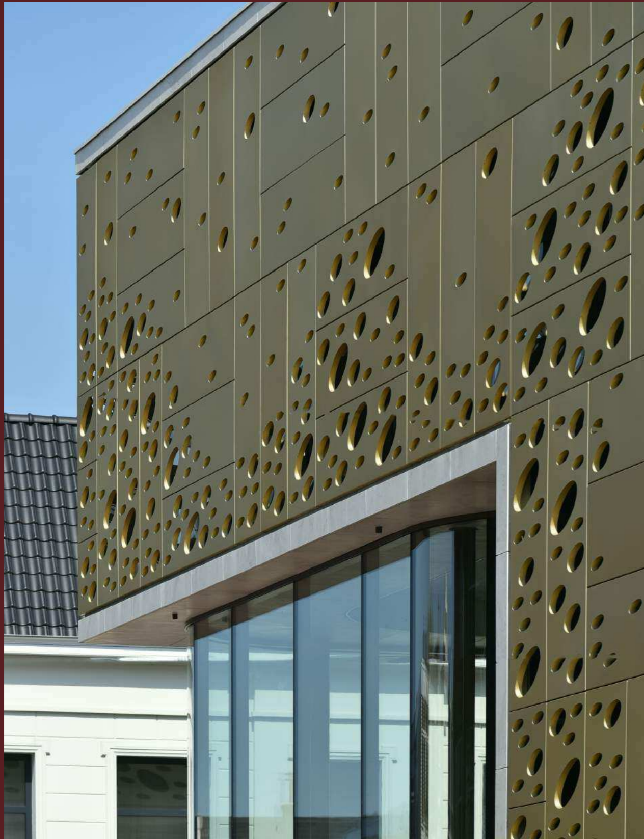
The six centimetres thick cassettes also have a structural function
